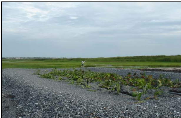
Tema Living Machine horizontal flow wetland at start up
